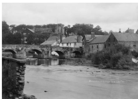
The main bridge into Brecon spans the river Usk. It was originally built in medieval times. That bridge was washed away by flooding in 1535. A new bridge was built in 1563 during the life of Elizabeth I [1533-1603]. In 1772 this second bridge was repaired and in 1794 it was widened. Its stone parapets were visible until the modernisation of the bridge in the 1970s, hid much of the original structure.
